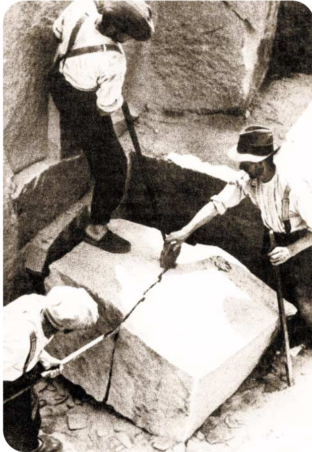
Spalten eines Granitblocks, trhlíny v žulovém bloku, cracks in a granite block
